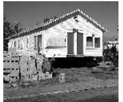
South L Street historic structure prepared for relocation
